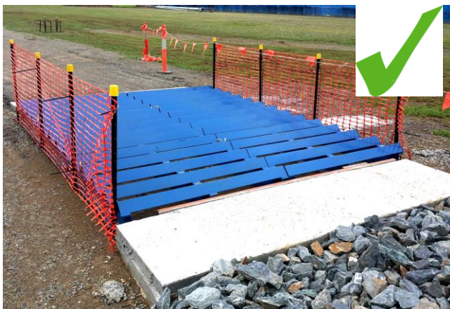
Rumble grid and rock pad in place on the Construction site exit.
