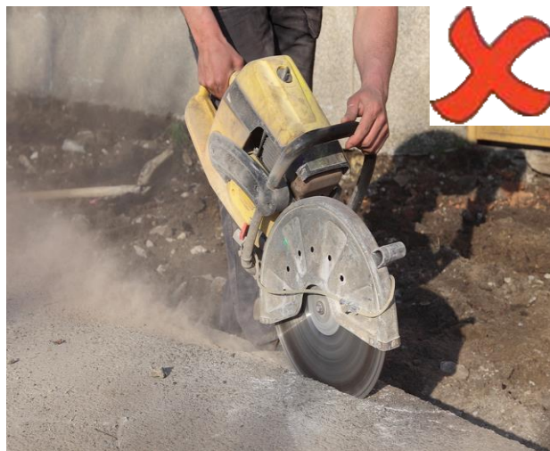
Concrete cutting with no dust suppression Controls.
