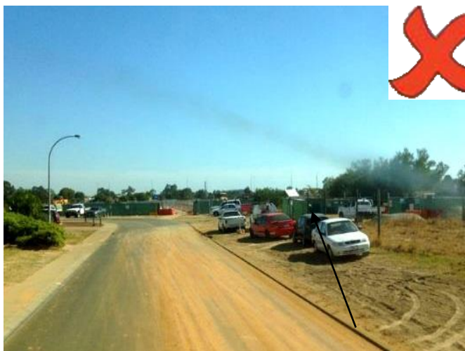
Dirt has been tracked extensively onto a public road. This can become airborne or enter stormwater drains.
